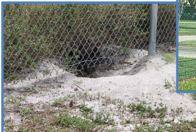
Photo 4-6 Perimeter fence breach
