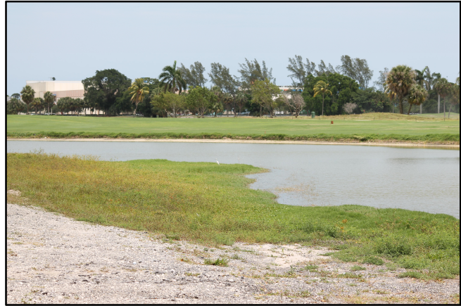
Photo 2. Stormwater pond at approach to Runway 24 at PMP.
