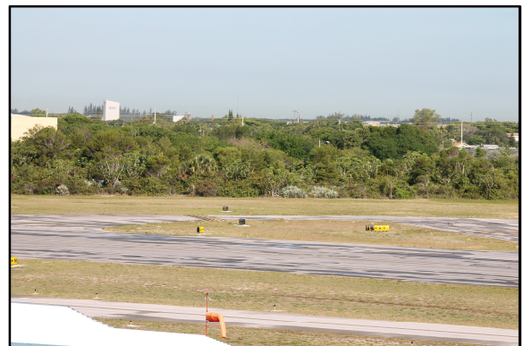
Photo 6. Wooded areas inside the perimeter fence at PMP.
