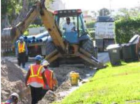
**Project Description:** This annual project is to continue the replacement of undersized galvanized water mains as well as unlined cast iron distribution mains throughout the City.
