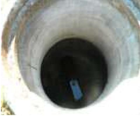
**Project Description:** This project involves the rehabilitation of deteriorated brick manholes located throughout the City. Rehabilitation consists of covering the interior surfaces with an adhesive, non-permeable material. 58 manholes have already been relined in FY 2015. Citywide there are 4,400 manholes.
