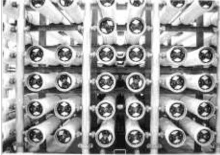
**Project Description:** This ongoing project consists of replacing the membrane elements (filters) when needed. The membrane elements are used to purify water to make it potable and requires replacement every 5 years. All filters were replaced in FY 2016. Funding will be budgeted over a multi-year period to provide for full replacement.
