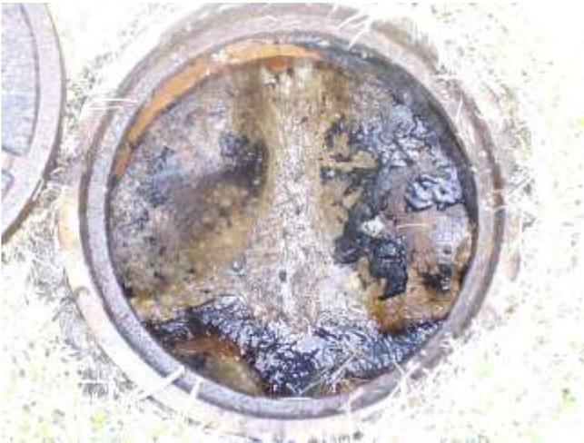
**Project Description:** This project involves the rehabilitation of deteriorated brick manholes located throughout the City. Rehabilitation consists of covering the interior surfaces with an adhesive, non-permeable material. 108 manholes were lined in FY15 and FY16. Citywide there are 4,400 manholes.
