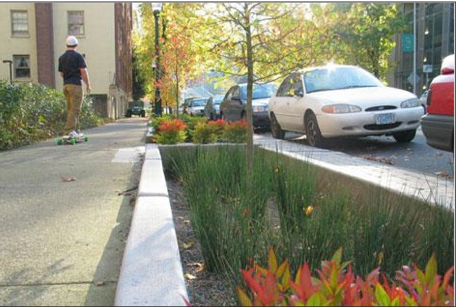
Green street bio-filtration systems can be incorporated between walk and bike lanes to gather, retain and treat stormwater if the local water table and grading can support these techniques.
