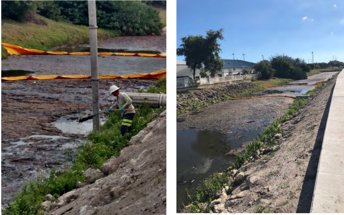
Figure 7: Floating material removed accumulated by the floating curtains and removed from site.
