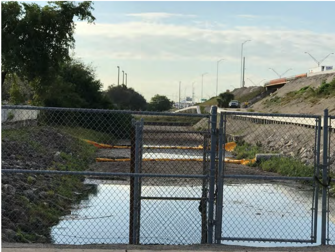
Figure 6: Floating material removed accumulated by the floating turbidity curtains and removed from site.
